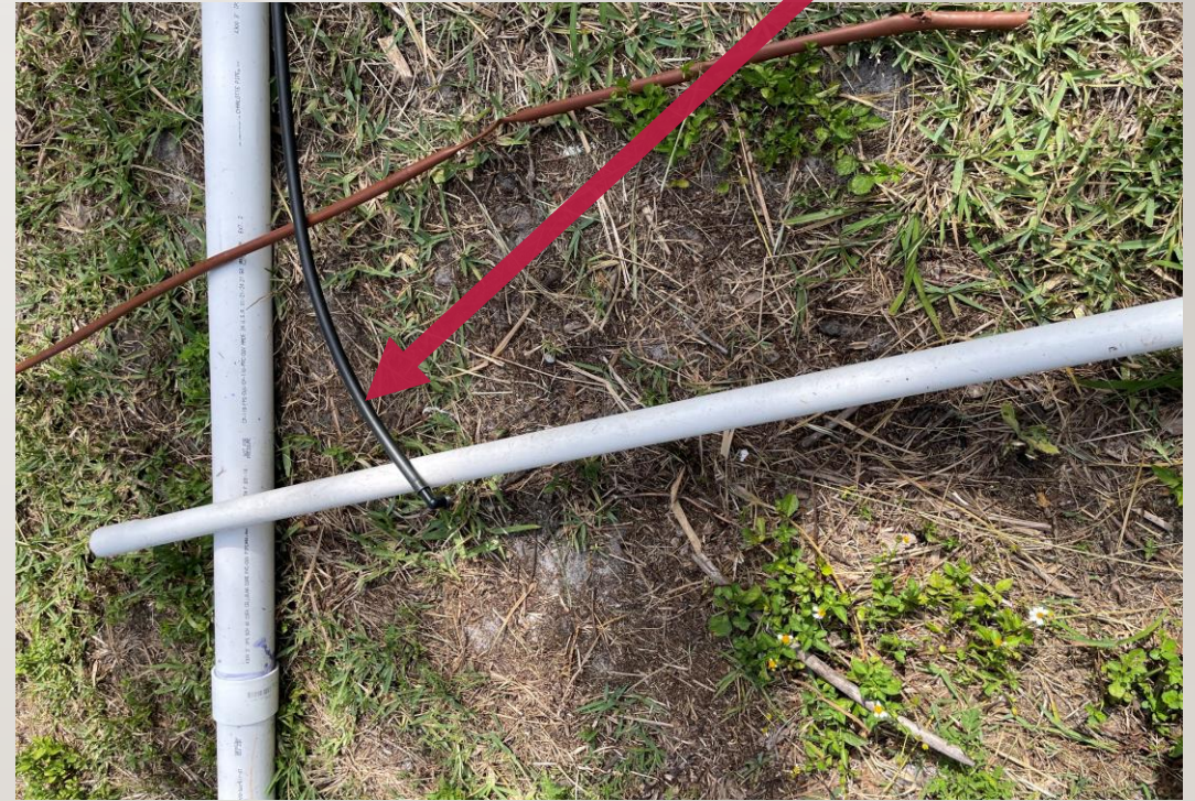
Connection from PCV to drip line-funny pipe
